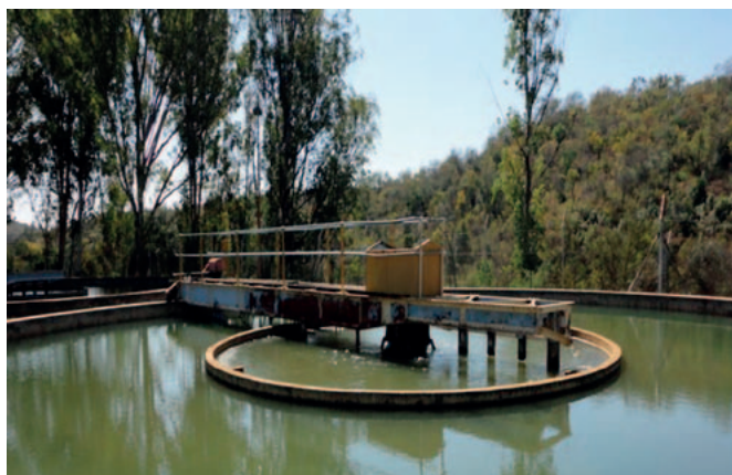
FIGURE 8: Primary Clarifier at Ncema, which is in need of rehabilitation.
