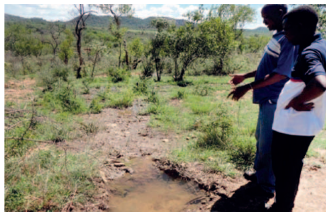
FIGURE 9: Leakages at the Inyankuni-Ncema Pipeline result in localised flooding.
